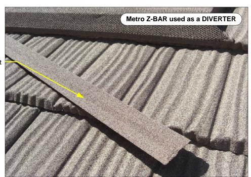
Metro (Small) Z-Bar Metal cut to fit across the front face of the SMART-Vent approximately 43inches long
